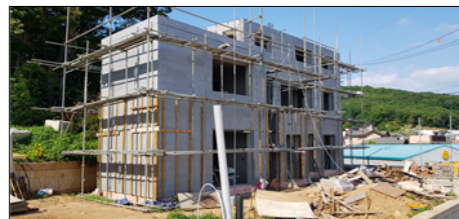
| EZBlock Construction Example
