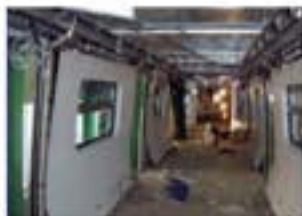
Inside Panel Installation
