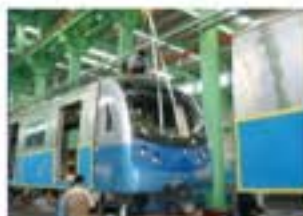
Driving Cab Module Installation
